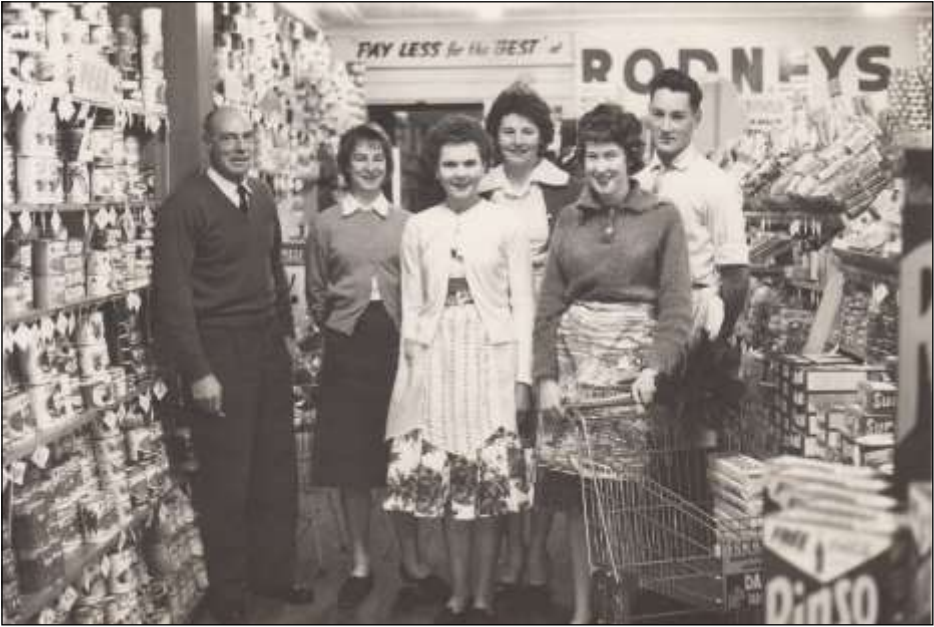
Staff Photo. Rodney's Grocery Store, 180-186 Argyle Street, (former Haffenden and Henderson building) opposite the Crown Hotel. Steve Cushing (Manager), Rhonda Chipperfield, Barbara Toovey, Joy Dunk (later Riley), Patricia Green, Wayne Taylor. (Camden Images)
